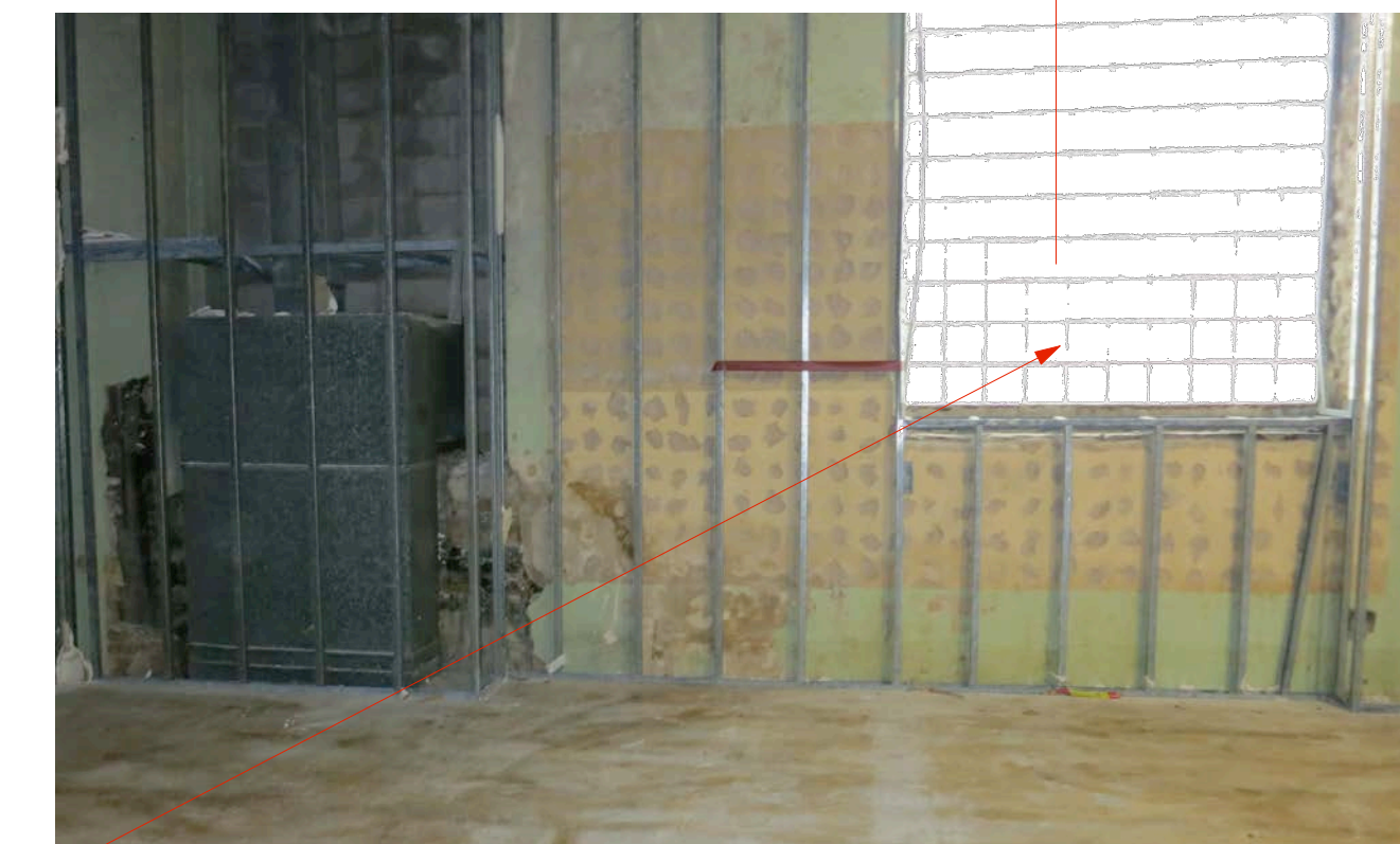
NORWOOD TOWER - GLASS BLOCK FILLED OPENING
