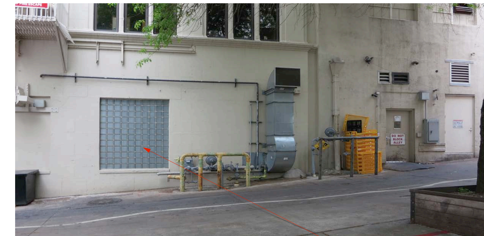
NORWOOD TOWER ALLEY - NORTH SECTION
