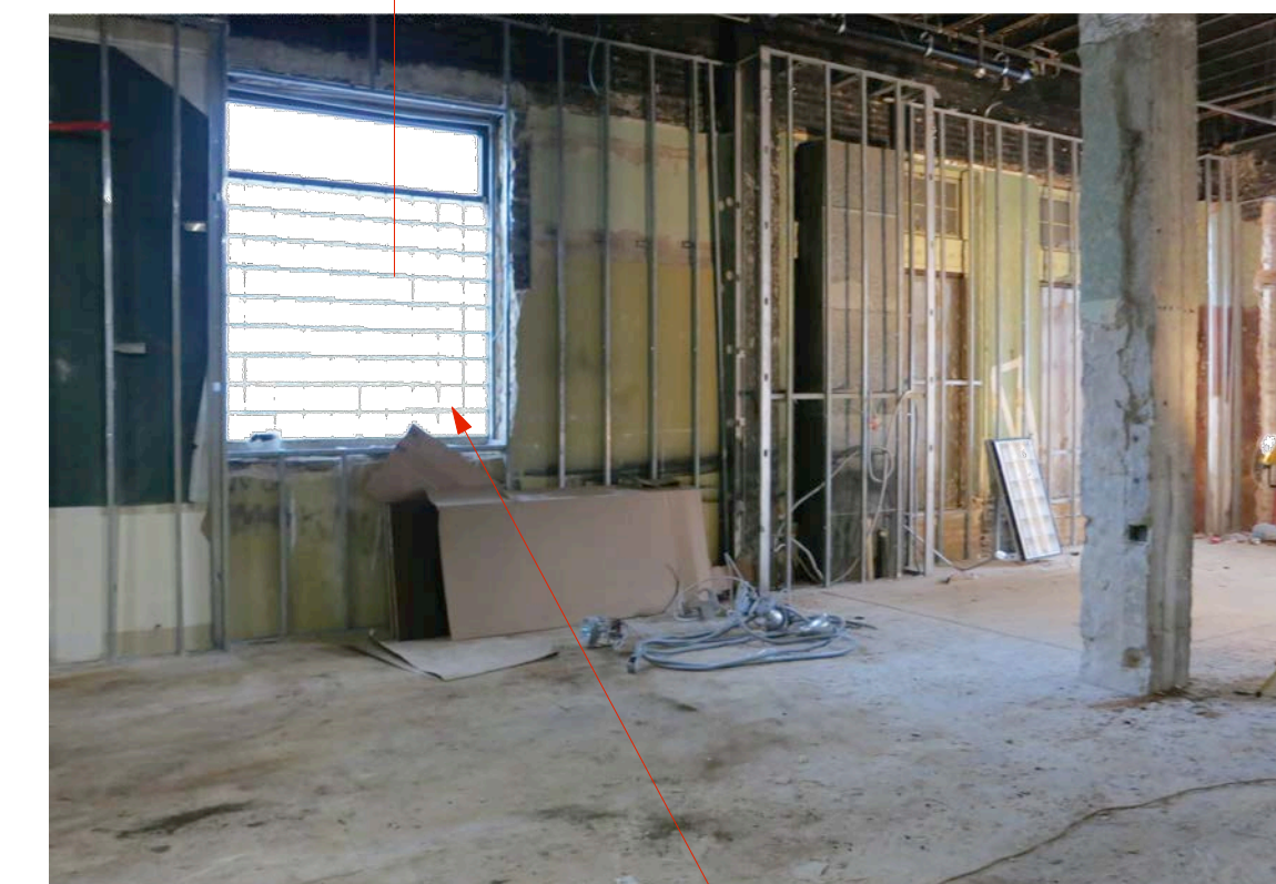
NORWOOD TOWER - GLASS BLOCK AND CLEAR GLASS FILLED OPENING
