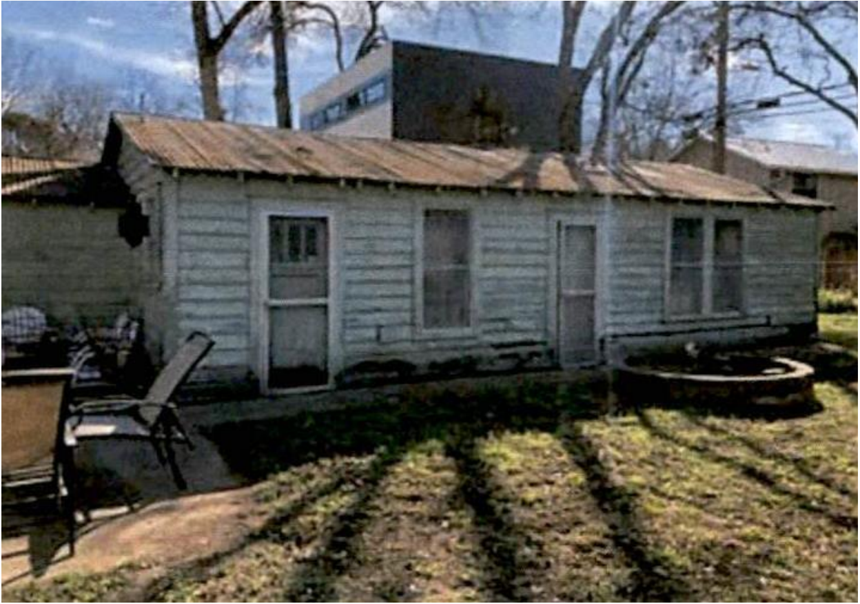
Existing garage building to be removed pursuant to this proposal.
