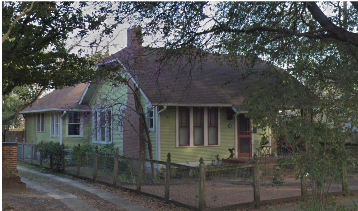
Primary (west) wall of 3803 Avenue H. Source: Google Street View, February 2019.
