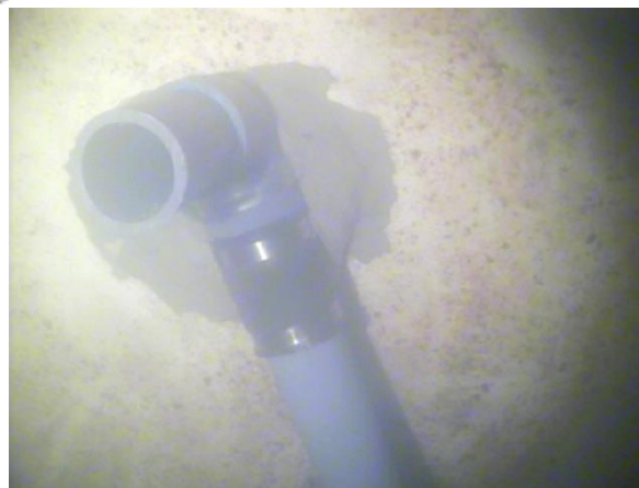
Chemical feed line discharge
