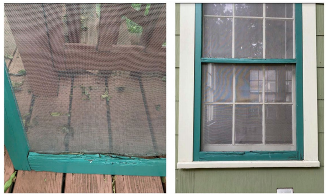
Representative Example of Screen Rotting
