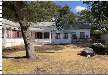
South façade at porch and addition Note: Porch windows are non-historic Porch to be rebuilt in similar configuration with all new windows Variances from current configuration provided to allow suitable porch roof flashing to historic east wall
