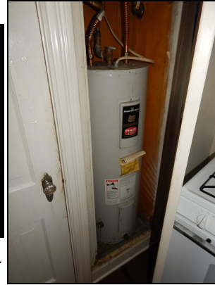
Down unit: 30 gal, 4500 watt unit.
