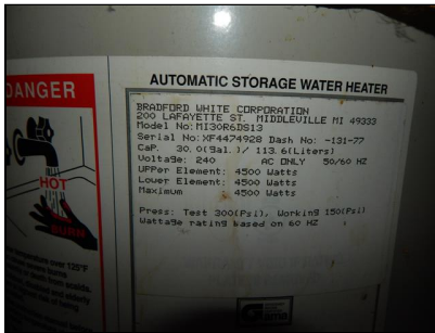
Upstairs unit: 30 gal, 4500 watt unit.
