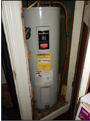
Down unit: 30 gal, 4500 watt unit.
