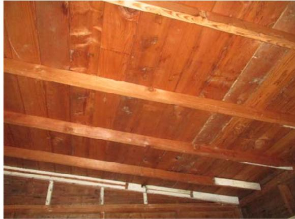
From the exterior of the addition we were able to observe that an elevated wooden floor framing system bears on a concrete slab. The photograph at lower left documents this framing pattern, as well as the deterioration of the sole plate for the exterior wall. The photograph at lower right is in the same general area, but a broader perspective. This photograph indicates that the water damage (rot) continues up the wall to the siding and presumably to the wall framing.
