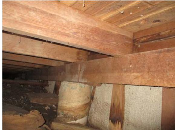
At least one of the concrete block piers is not in contact with the beam (photograph at lower left). The only water damage to the wooden subfloor framing that we observed in the accessible areas was at the bathtub. Refer to the photograph at lower right.
