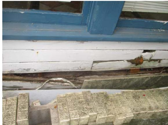
For this type of wall construction the building code (International Residential Code) requires a minimum of six inches from grade to the top of the foundation to prevent surface water intrusion. This clearance was not provided. The result is extensive deterioration of the exterior wooden framing.
