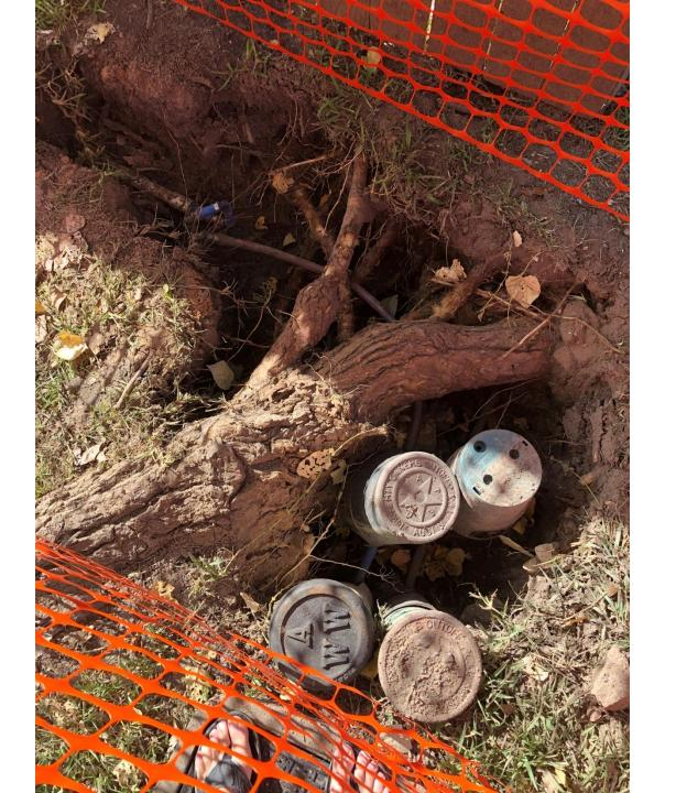
Root was excavated by Austin Water – Roots are clearly destroying pipes.
