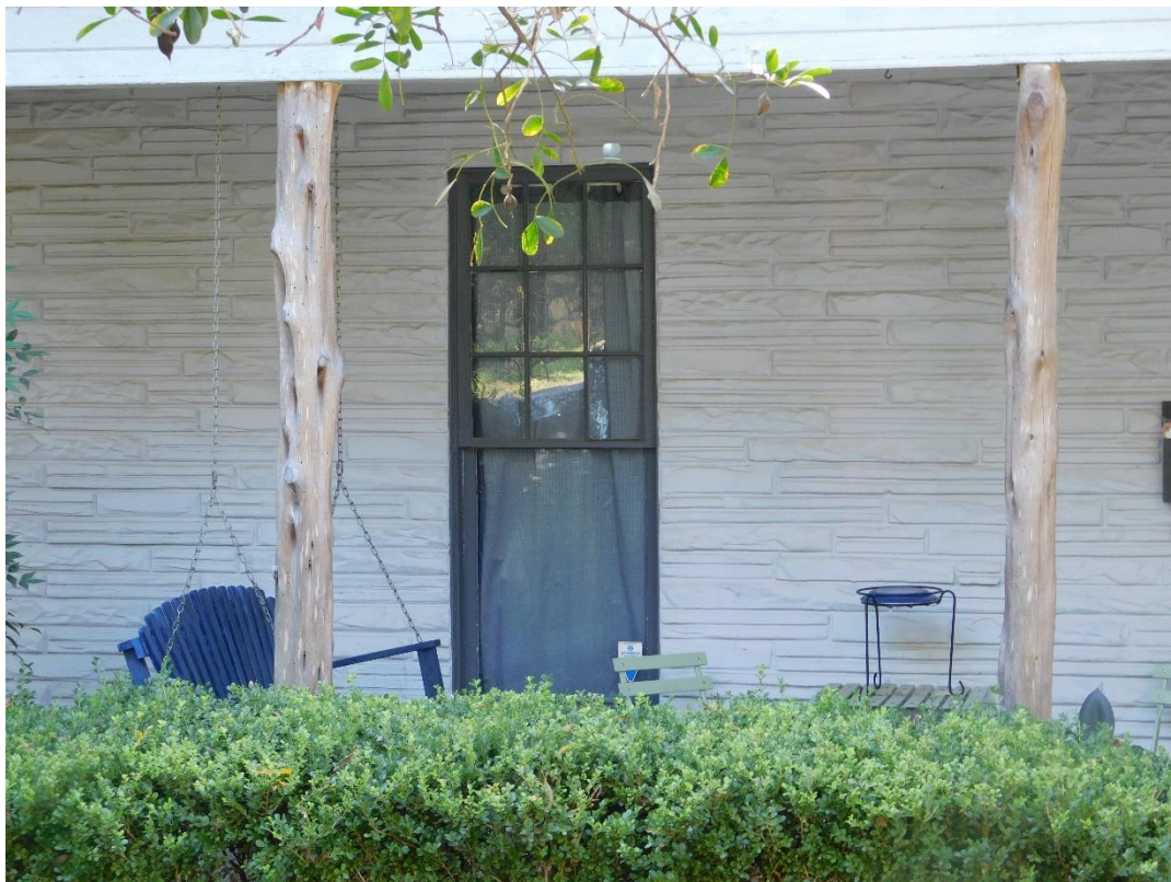
Detail of permastone siding, wood porch posts, and 9:1 window
