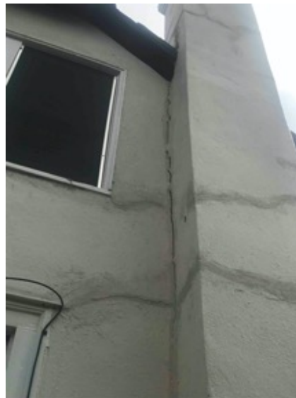
CRACK AT CHIMNEY
