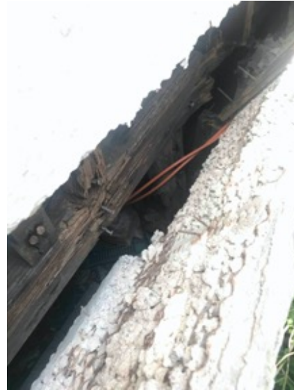
ROTTING BEAMS
