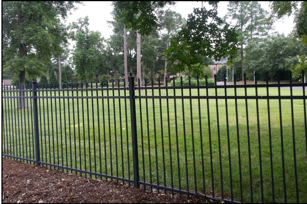
If this fence is less than 6 feet in height, and horizontal members are less than 45 inches apart, it could be in compliance if the finials are spaced no less than 6 inches apart.
