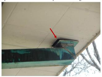
The downspout(s) should discharge water at least five (5) feet from the house. Storm water should be encouraged to flow away from the building at the point of discharge. Ramps or extension tubes are recommended.
