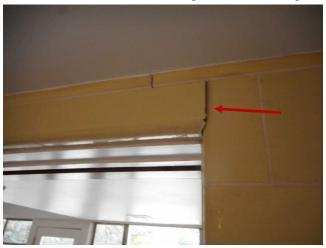
Larger than typical cracks were noted in the master bedroom. This condition could indicate greater than normal movement within the structure and potential structural problems. Further investigation may be necessary.
