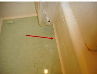
The tile shower stall requires repair in the master bathroom. Loose or damaged tile, grout and caulk should be repaired or replaced as necessary. Any damage to the wall behind the tile should also be repaired (if necessary). Further investigation may reveal the need to rebuild a portion of the shower stall.
