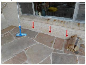
Steel lintels were not installed over some of the windows on the home. This does not comply with IRC code for home construction.
