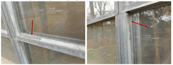
Safety glass etchings were not observed on the glass within the windows next to exterior doors. This glass is required for windows close to the floor or in hazardous locations and is generally identified by an etching in the corner of the glass pane.
