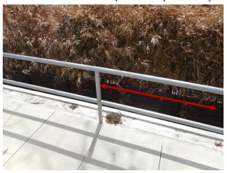
The height of the rooftop railing may not be sufficient to prevent a person from toppling over the railing. It is recommended that this condition be repaired for improved safety.
