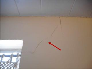
Larger than typical cracks were noted in the south east bedroom. This condition could indicate greater than normal movement within the structure and potential structural problems. Further investigation may be necessary.
