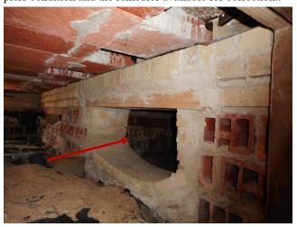
Substantial foundation cracking was observed in the front entry. This implies that structural movement of the building has occurred. The rate of movement cannot be predicted during a one-time inspection. A structural engineer should be consulted to further evaluate this condition and the remedies available for correction.
