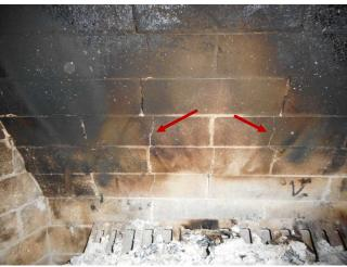
A vermin screen should be installed on the chimney. The fireplace damper does not operate and requires repair.
