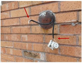
The exterior outlets on the roof and landscaping are not connected to a ground fault circuit interrupter (GFCI) circuit. Under current electrical standards, all of the exterior receptacles should be connected to a ground fault circuit interrupter (GFCI) circuit. *The lack of this outlet(s) is a recognized hazard*.
