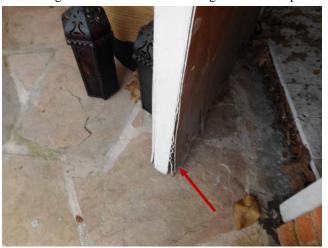
The doors to the kitchen pan try should be trimmed or adjusted as necessary to work properly.
