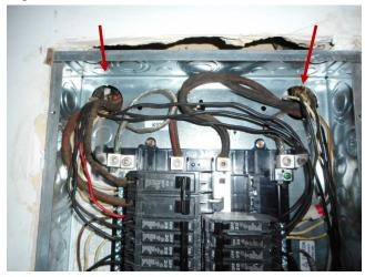
The sub panel should be sealed to the structure on the top and sides, leaving the bottom open. This will help prevent water penetration behind the panel.
