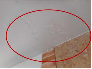
Larger than typical cracks were noted in the master bathroom. This condition could indicate greater than normal movement within the structure and potential structural problems. Further investigation may be necessary.
