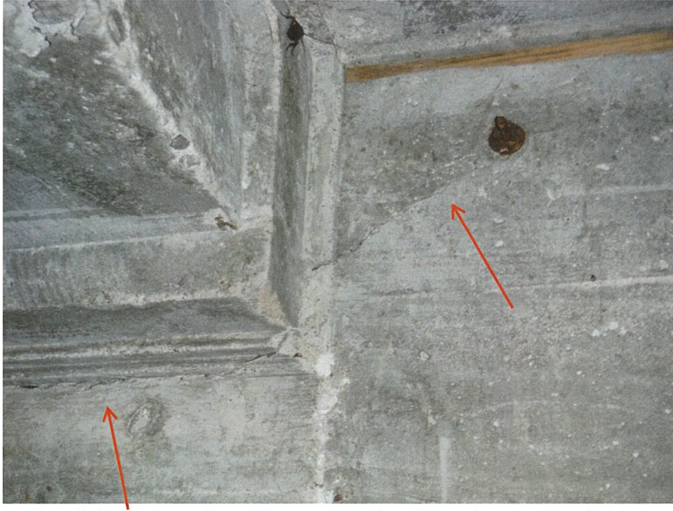
Figure B11 – Typical cracks in foundation wall at ends of middle beams at Fire Station No. 3
