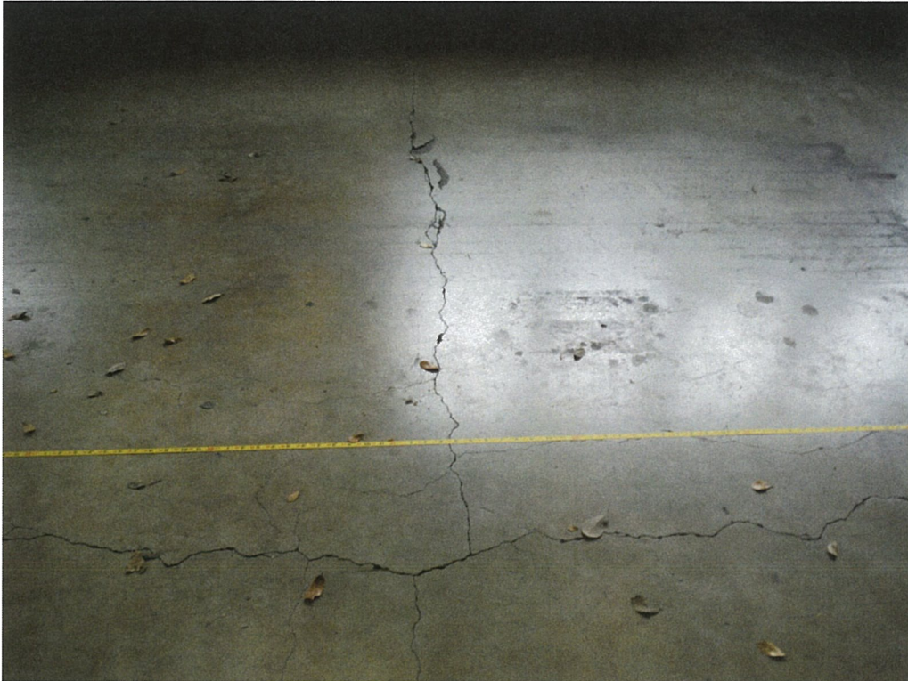
Figure B7 – Typical cracking in top of slab at Fire Station No. 3 garage
