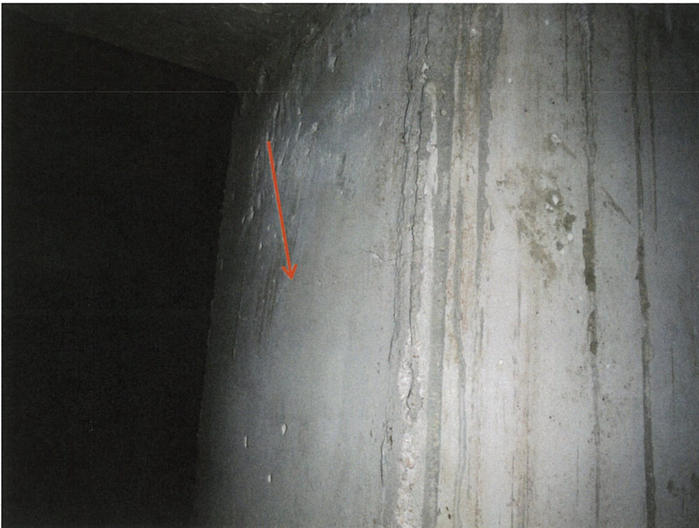
Figure B10 – Typical horizontal crack in column at Fire Station No. 3
