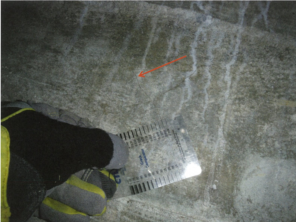
Figure B9 – Crack in west beam at north end of garage at Fire Station No. 3
