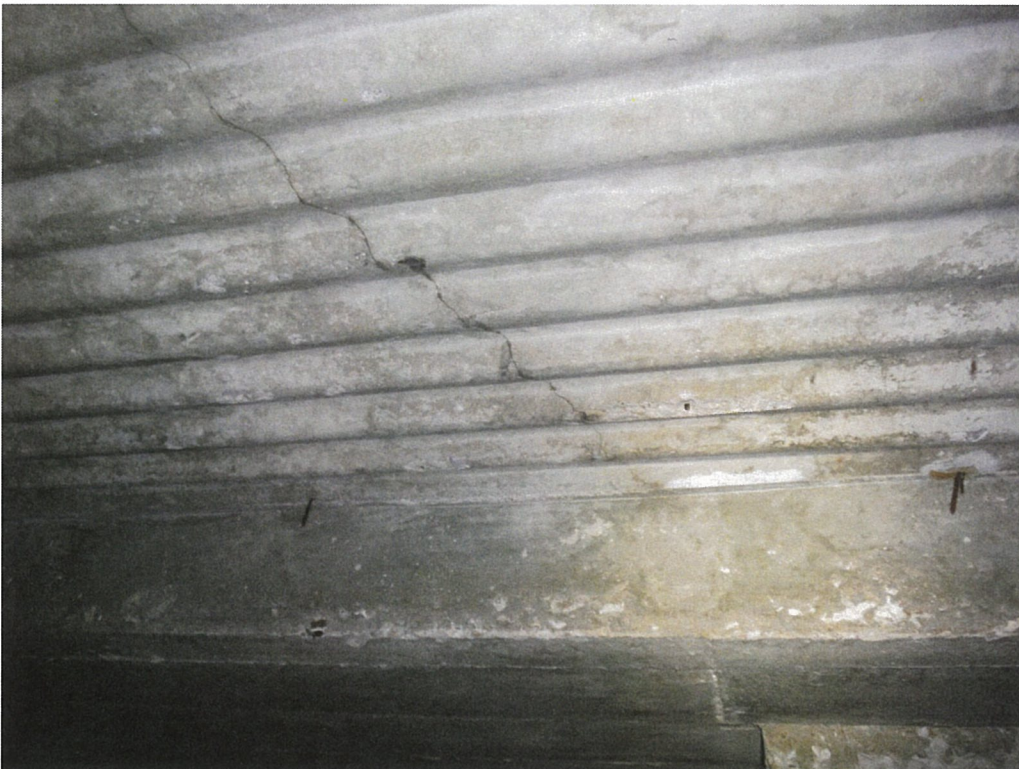
Figure B8 – Typical cracking in underside of slab at Fire Station No. 3 garage
