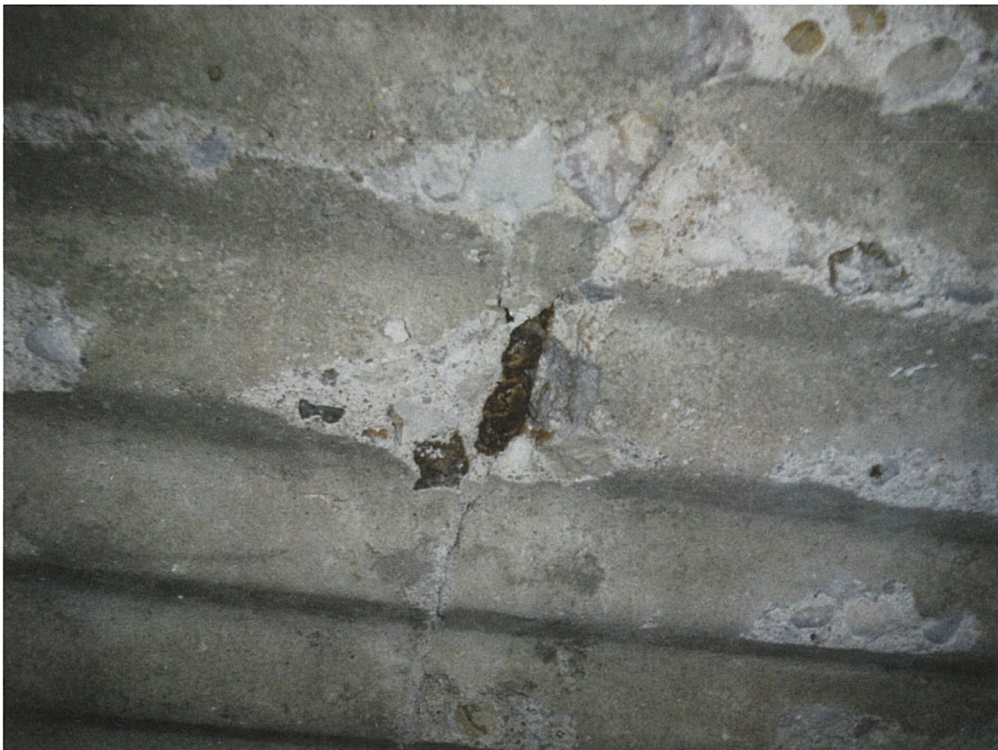
Figure B12 – Spalled concrete and corroded reinforcement at underside of slab at Fire Station No. 3
