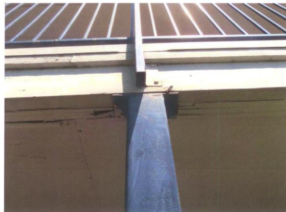
Photo 6 (BLDG 2): Top Plate Connection of Existing Steel Column
