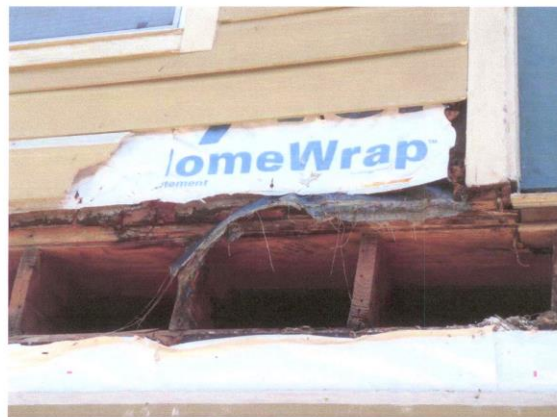
Photo 5 (BLDG 2): Existing Second Floor Framing Members
