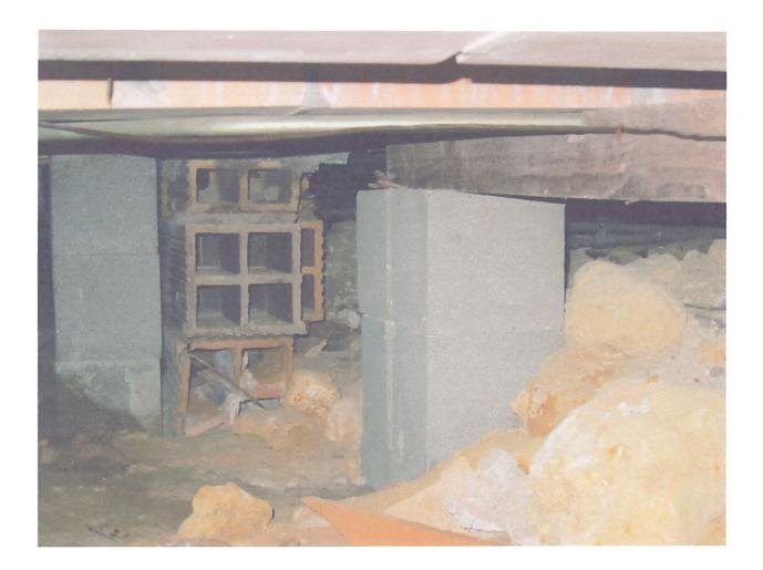
Another picture of crawl space below kitchen and dining room showing masonry supports of floor joists
