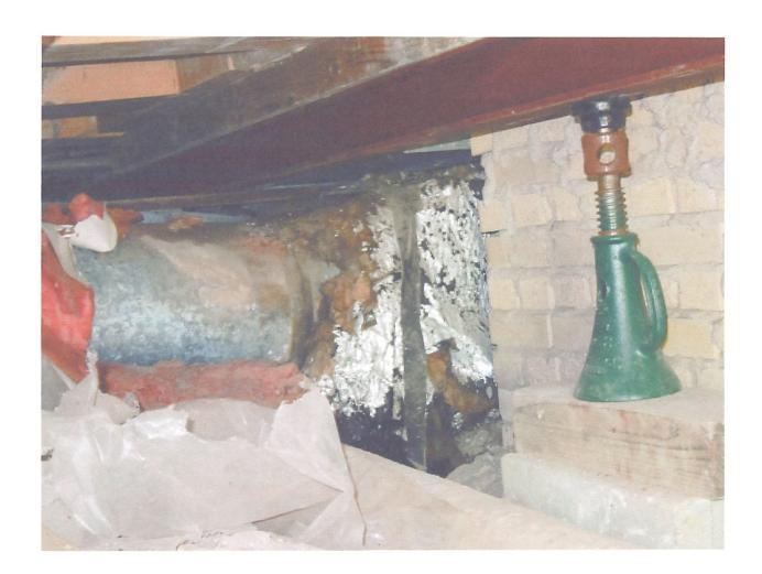
Picture of substructure below kitchen and dining room area showing jack remaining in place
