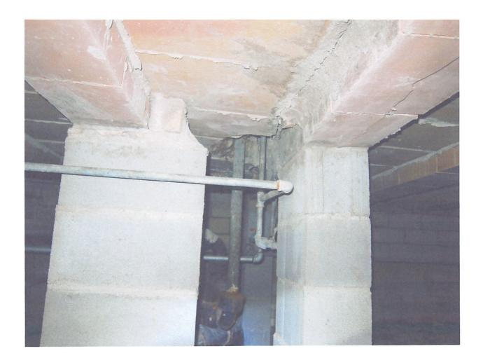
Area below room on west side of garage showing concrete masonry supports of floor joists, the installation of which was made prior to 1959
