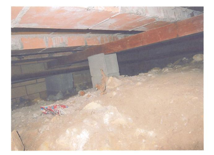
Area beneath dining room showing masonry block installation supporting floor joists
