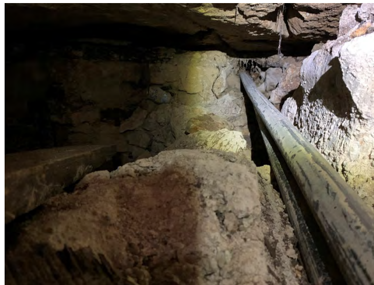
PHOTO 8 View of 2-inch-diameter buried steel piping running through cave next to WWL, facing north
