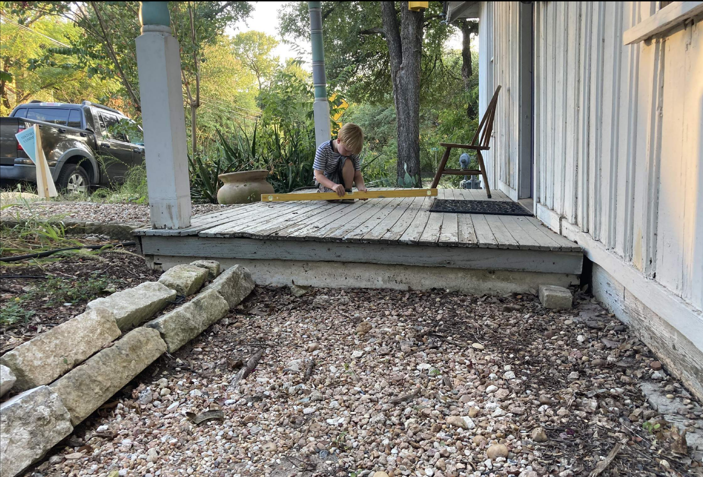
minor structural issues with original Juniper piers
