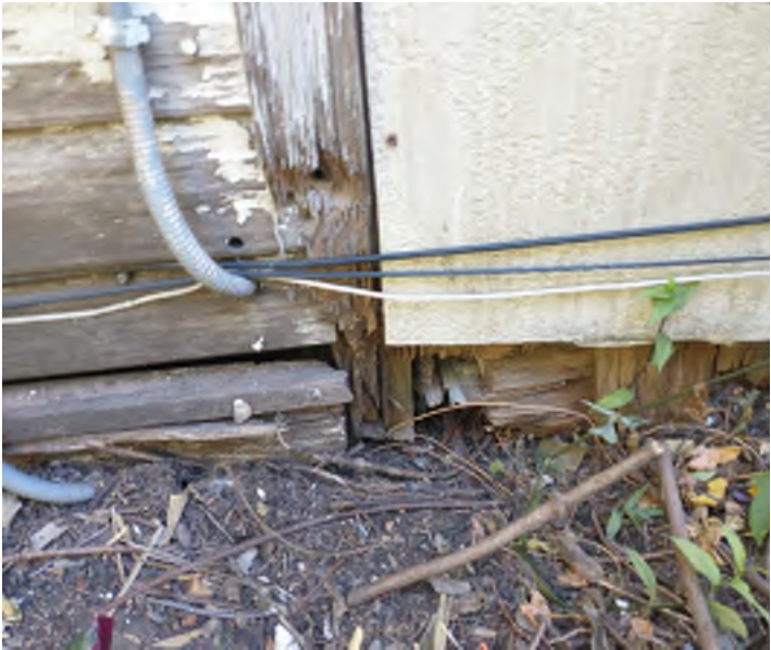
Rotted Wood in Contact with Ground
