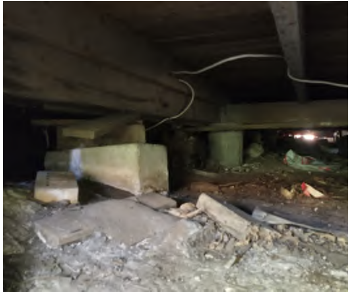
Foundation Crawlspace – Block and Conc Pier
