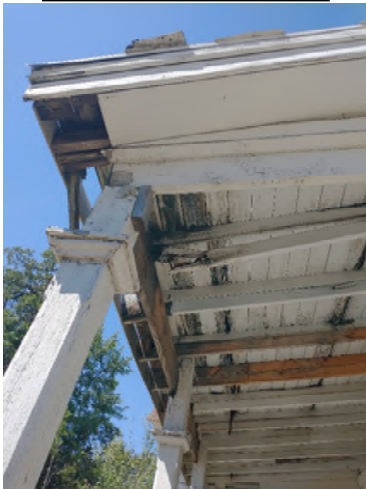
Rotted and Damaged Roof Framing
