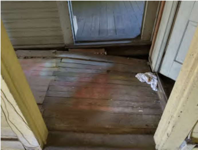
High Levels of Foundation Movement
