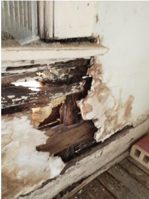
Water Damaged Studs and Sheathing
