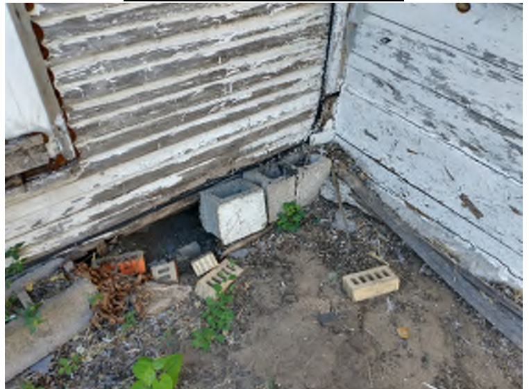
Water Damaged Studs and Sheathing
