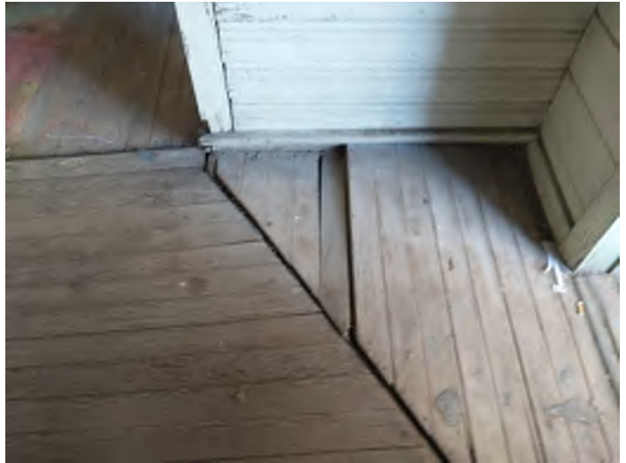
High Levels of Foundation Movement
