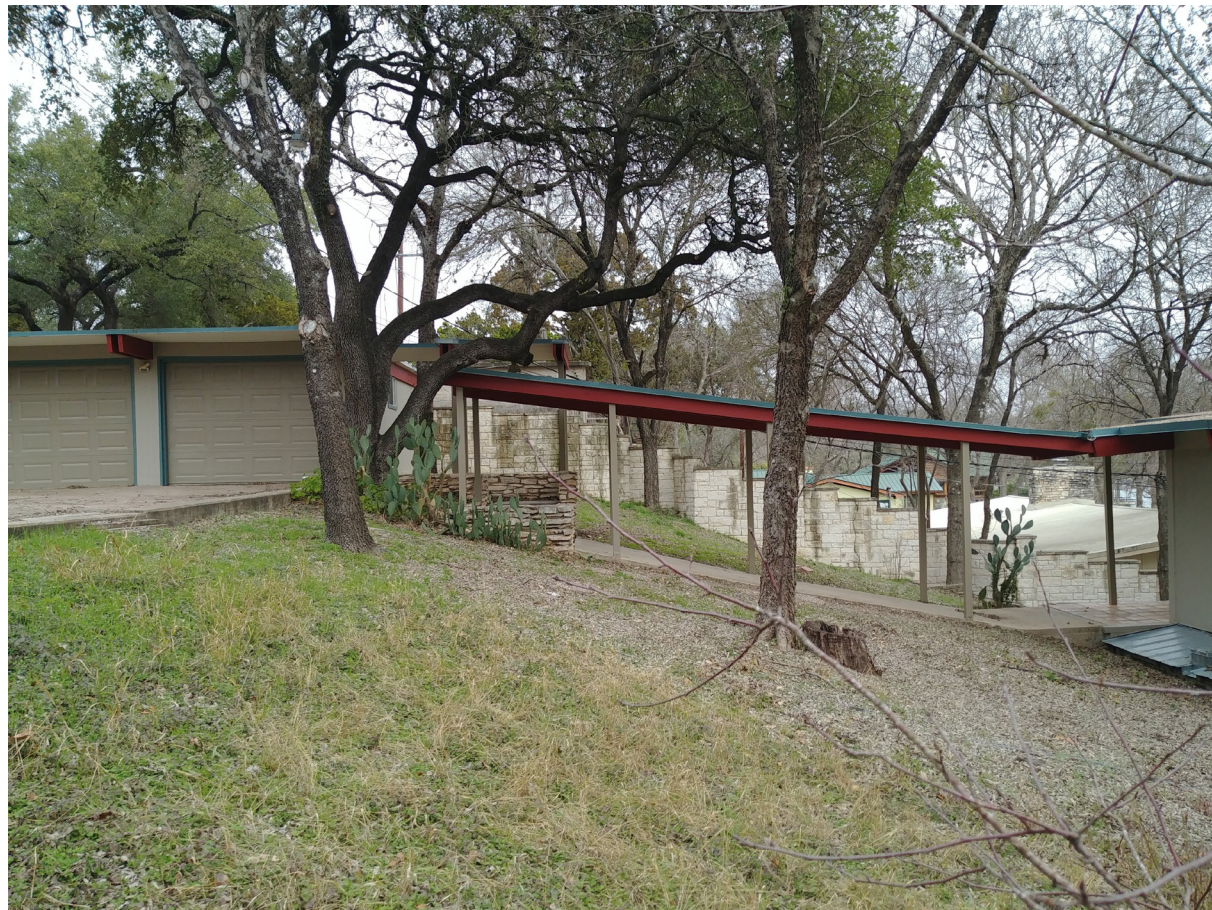
EXISTING ACCESS FROM GARAGE IS STEEPLY SLOPED WITH NO RAILING
