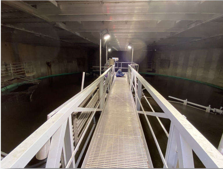
Rehabilitated Gravity Thickener
