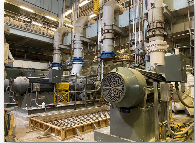
Replacement of Main Plant Lift Station Pumps
