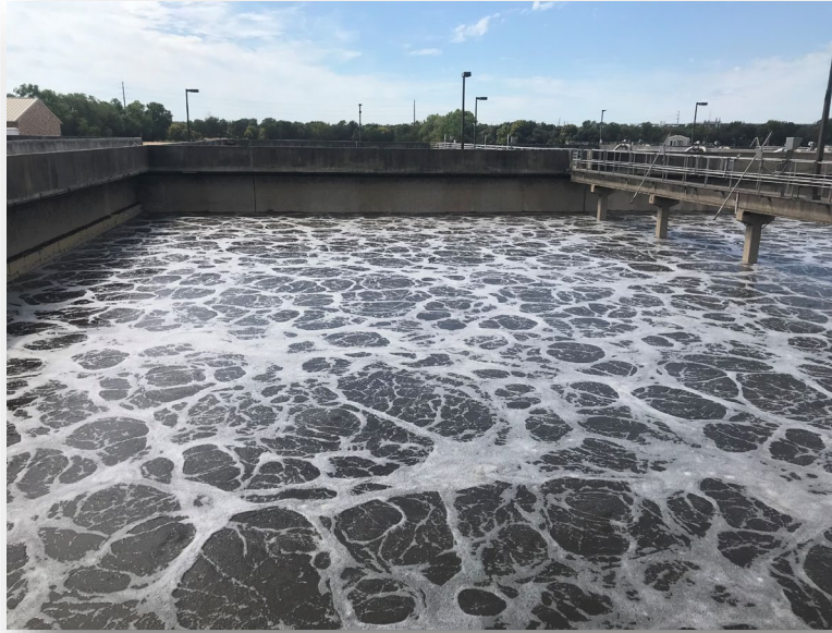
New Diffusers in all Aeration Basins
