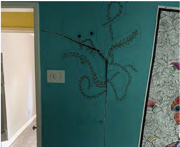
Cracks and Shifting
