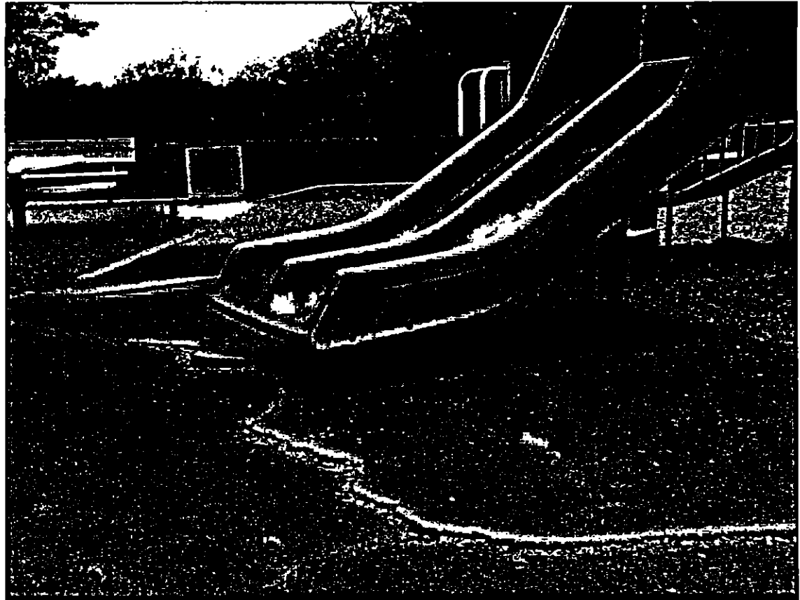
Example of failed rubber safety surface which had to be replaced.
