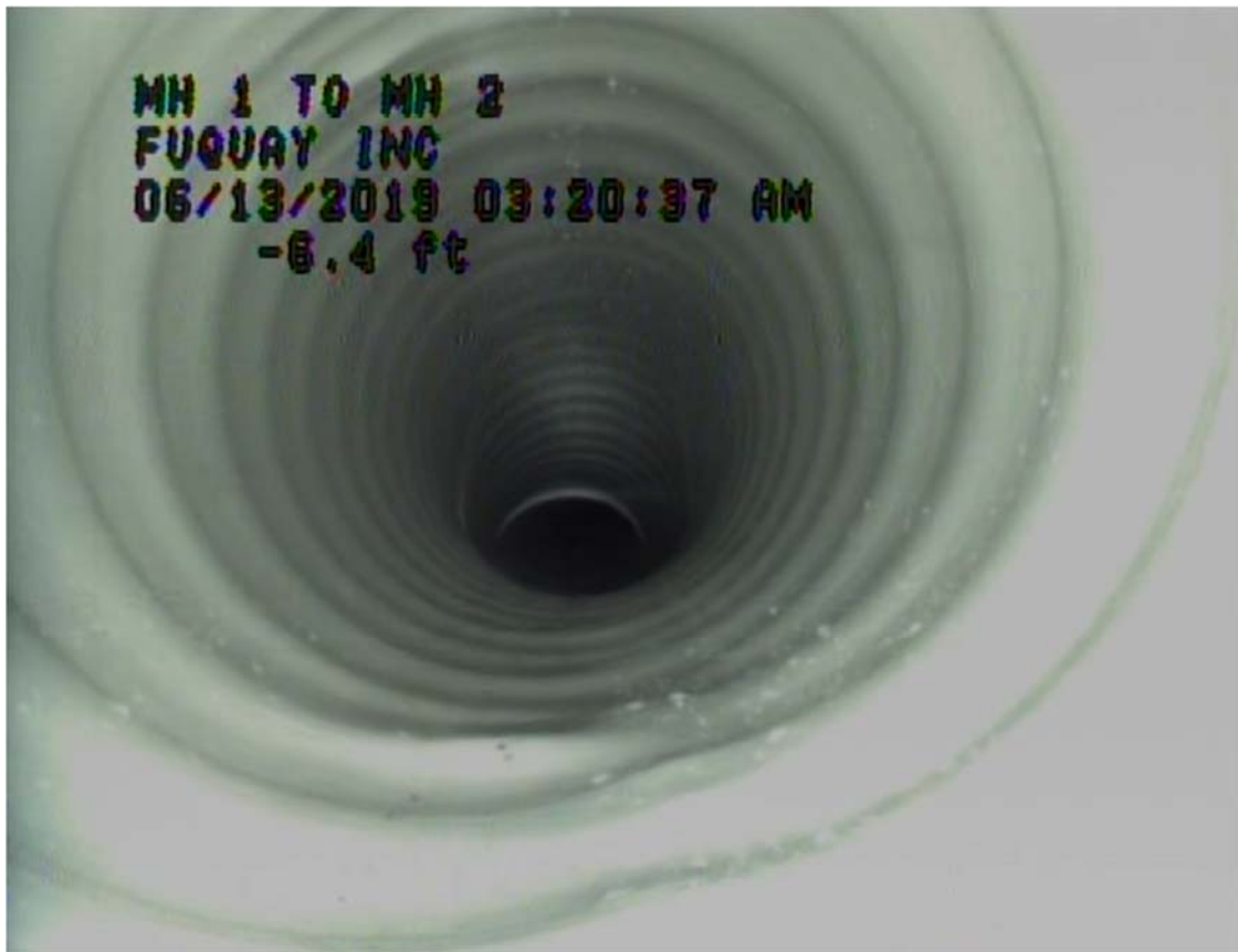
Photograph #5 – Rehabilitated Storm Drain Pipe
