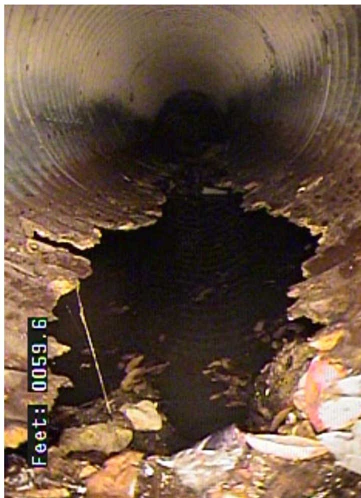
Photograph #4 – Corrugated Metal Pipe, Bottom Gone
