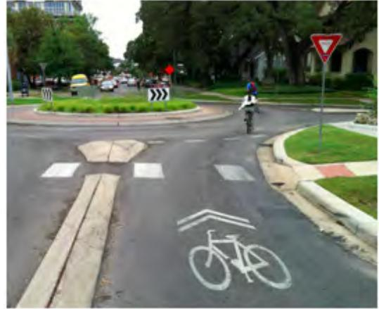
measures to discourage through trips by motor vehicles and create safe, convenient bicycle crossings of busy arterial streets (NACTO Urban Bikeway Design Guide, 2014).
