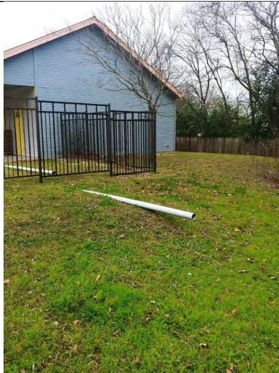
Photo 6: Eastern portion of property showing a pipe which conveys roof drainage to green space which ultimately drains to the storm water retention pond in the northwest portion of the subject property.
