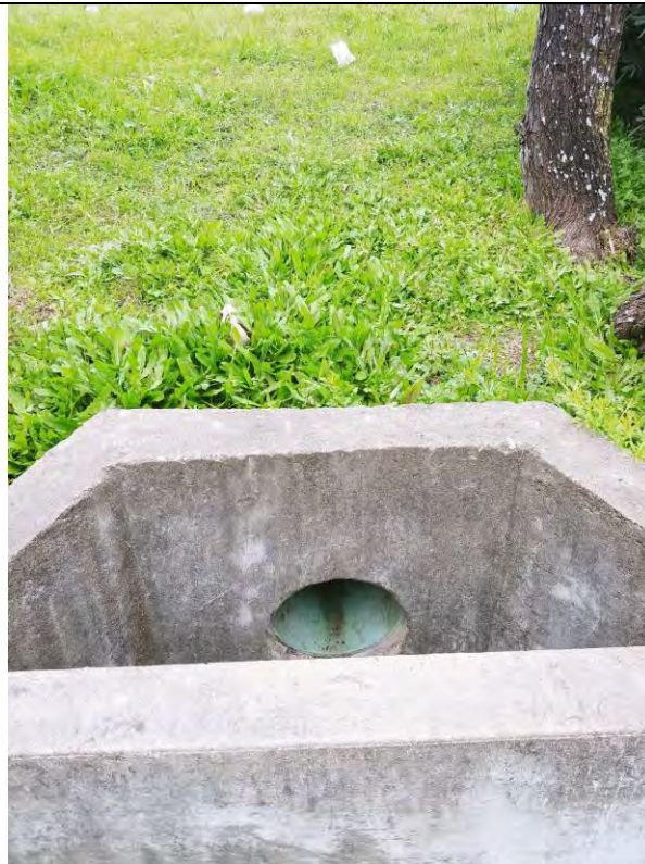
Photo 10: Storm water inlet at the west end of the storm water retention pond (in the northwest portion of the subject property between Montopolis Drive and the building).
