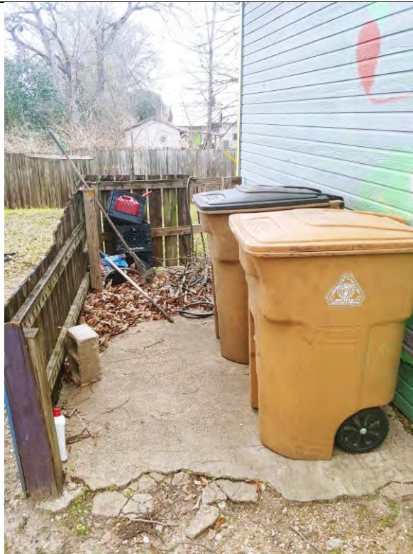
Photo 12: Trash bins on small concrete pad at the northern portion of the building.
