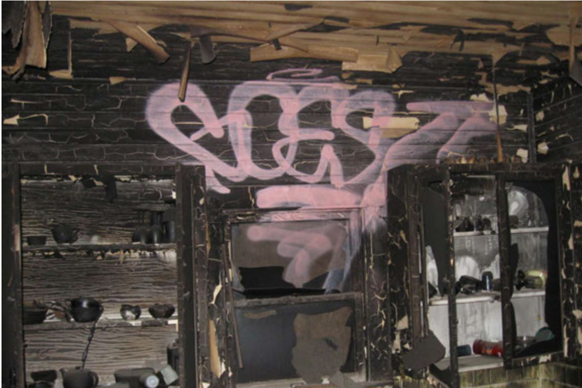
Photo 9 – This photo shows the fire damaged wall of the kitchen inside the house.
