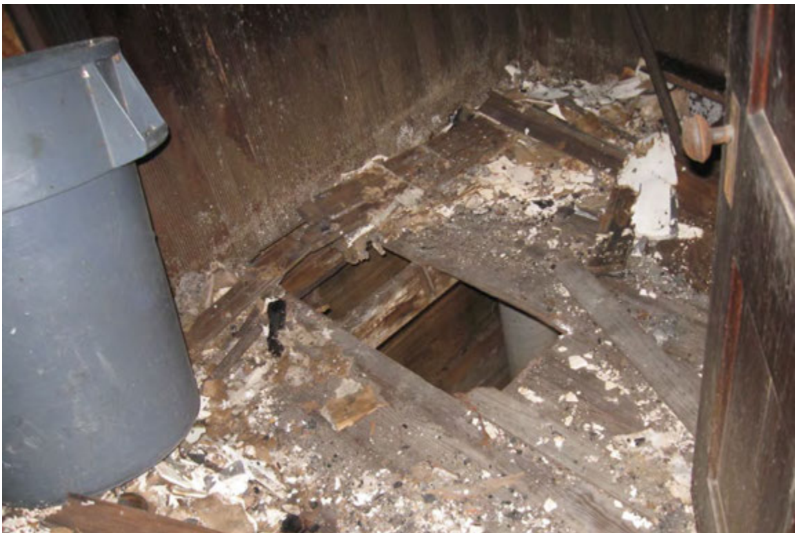
Photo 10 – This photo shows the debris covered floor and a hole to the crawl-space.
