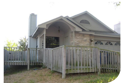
Home repair – accessibility modifications
