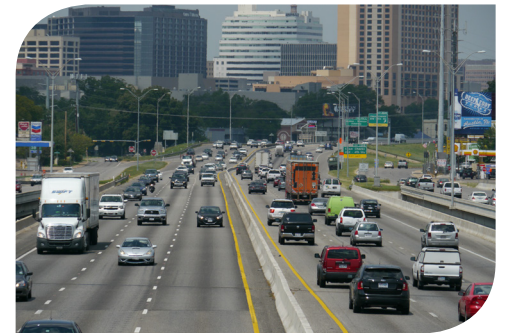
Interstate Highway 35 (IH-35)
