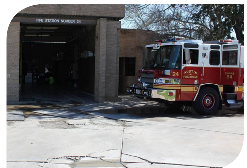
Fire station driveway replacements
