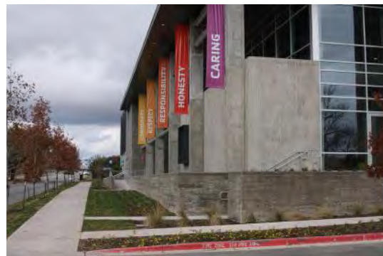
The YMCA/North Austin Recreation Center, completed in 2012, was built as a partnership between the Parks and Recreation Department and the YMCA.
