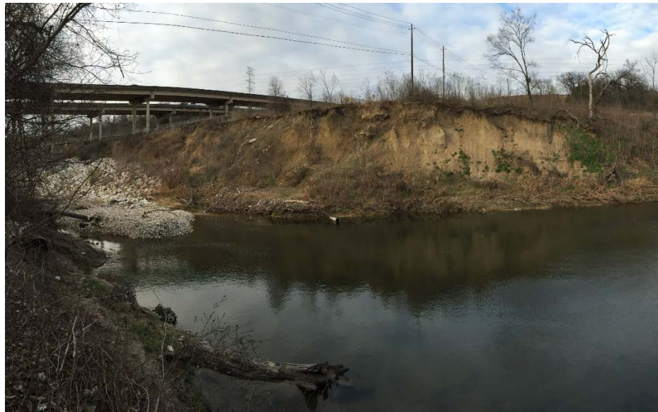
Boggy Creek – Hwy 183 to Delwau Ln Channel Stabilization
