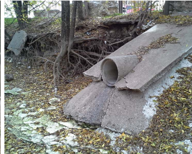
Little Walnut Creek – Jamestown Dr Stream Stabilization and Storm Drain Improvements
