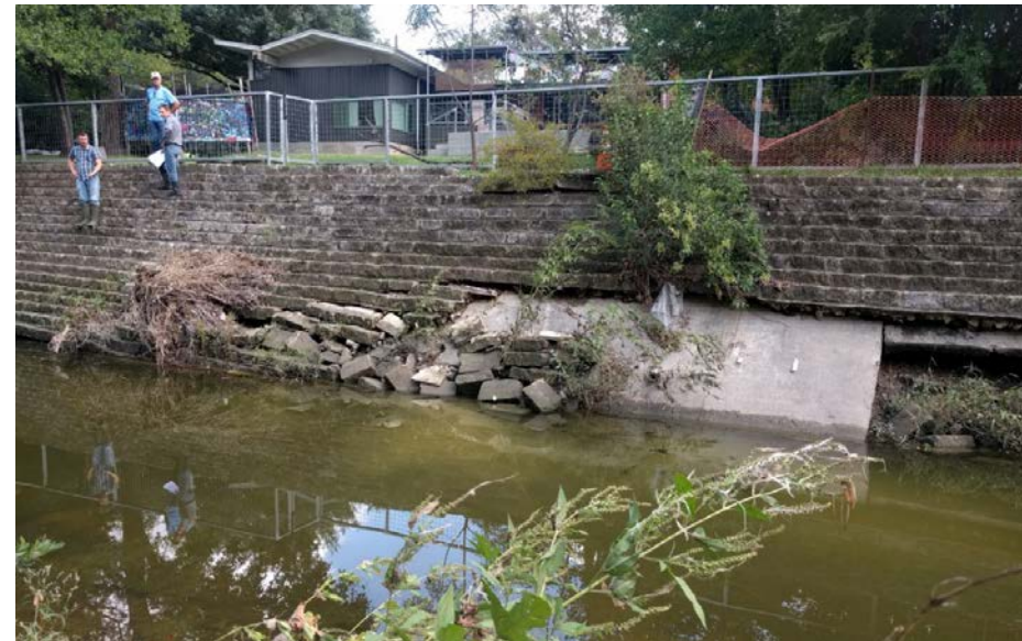
Citywide – General Stormwater Infrastructure Maintenance Projects Parent Account
