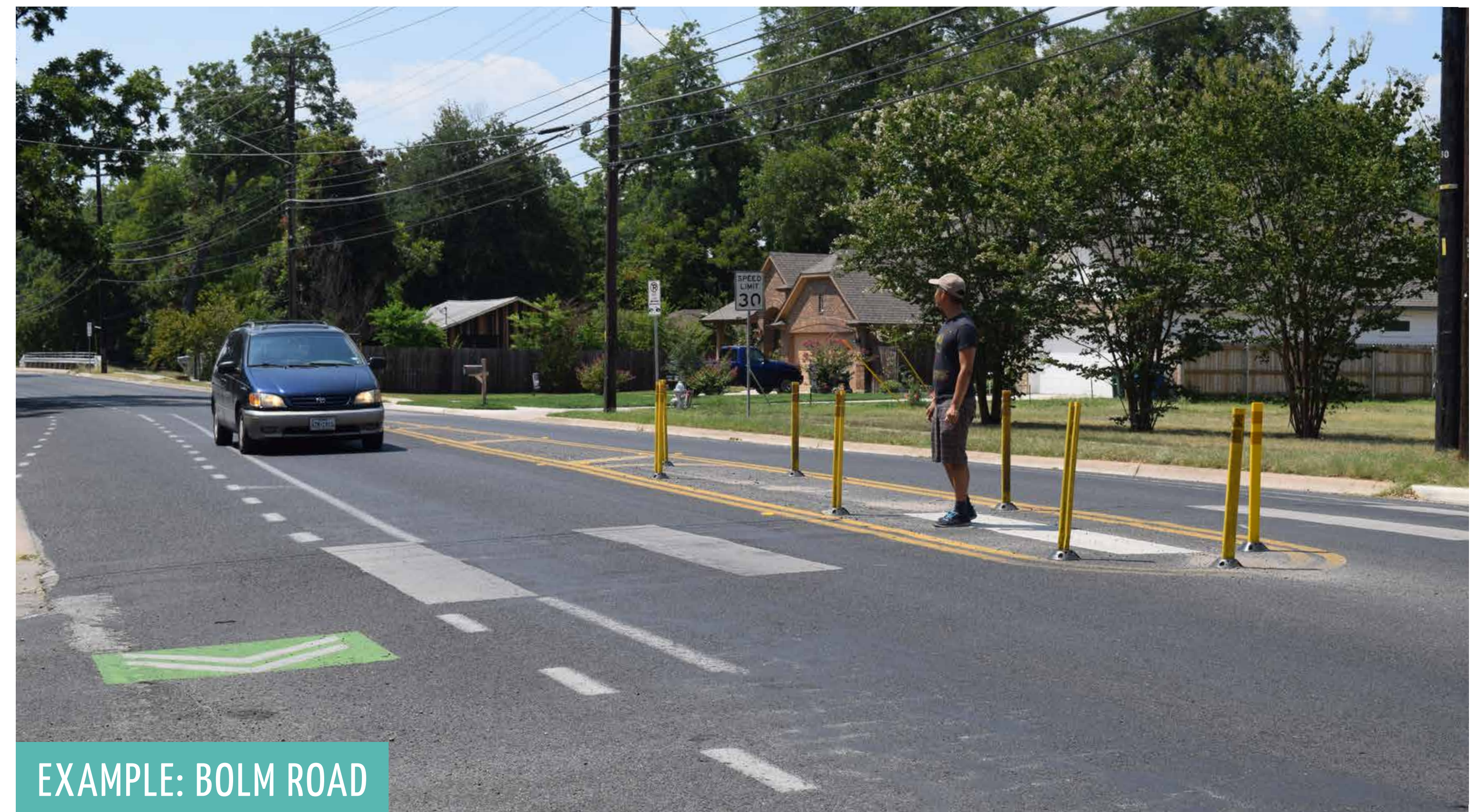
Example of a pedestrian crossing island constructed with flexible posts
