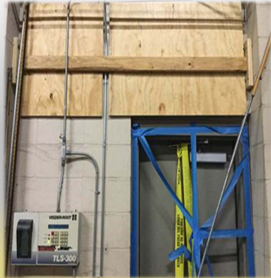
FIRE Station 32. Shoring of failing wall
