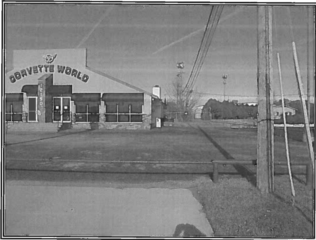
View of Subject Property west from Mopac Expressway
