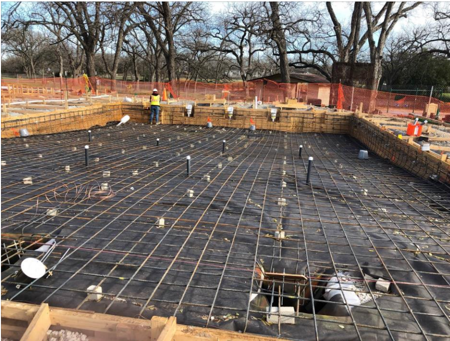
Activity pool rebar installation
