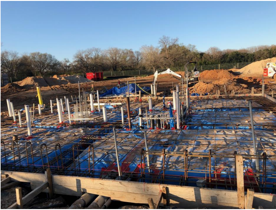
Pool bathhouse prepared for concrete pour
