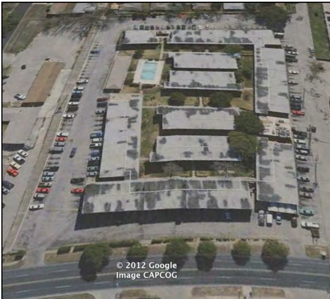
Sunnymeade Apartments at 501 E. Oltorf, April 2006, pre-demolition.
