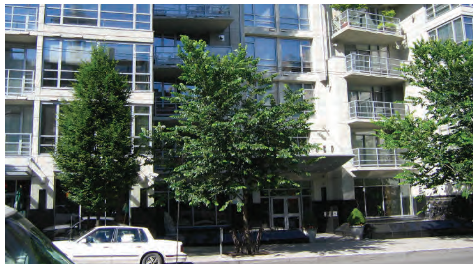
Figure 4.23 : Examples of Buildings Typical of the Commercial Mixed Use District
