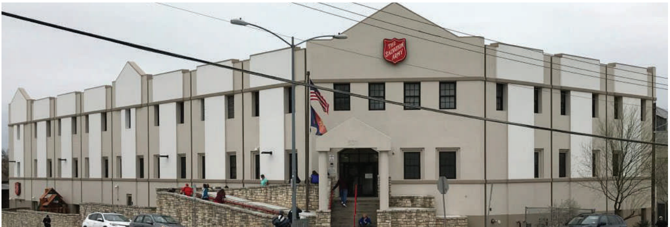
Project: Salvation Army Downtown Renovations Architect: O'Connell Robertson Scope: 84,000 SF shelter renovation
