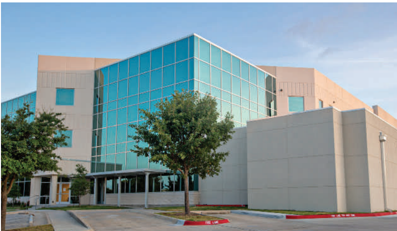
Project: Texas Oncology Renfert Vault Architect: RS&H Architecture Scope: 17,002 SF addition and remodel
