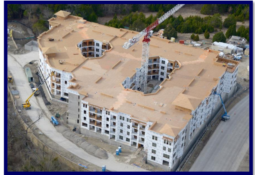
Florence at the Harbor Apartments, Rockwall (while Under Construction)
