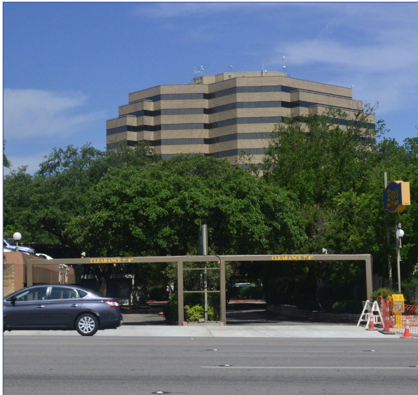
Figure 1-5: The City of Austin, in One Texas Center, is one of the largest employers in the South Central Waterfront.
