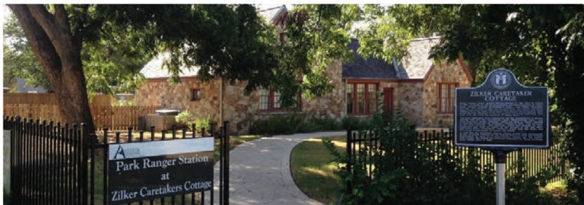
Zilker Caretaker's Cottage Restoration Winner of Preservation Texas 2018 Honor Award
