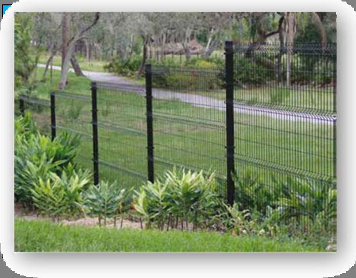
Proposed Steel Mesh Fence Height Varies: 4' ht. at Tree Court Overlook, 6' ht. All Remaining Areas.
