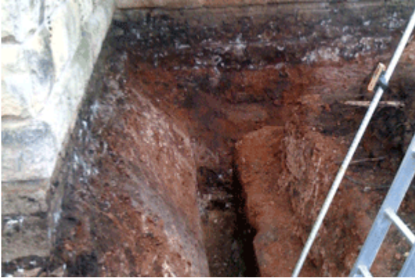
Stepped trench at southwest corner of building exposing foundation footing.
