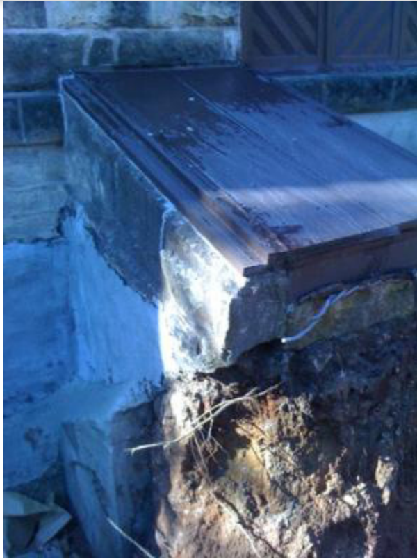
Underpinning of column
