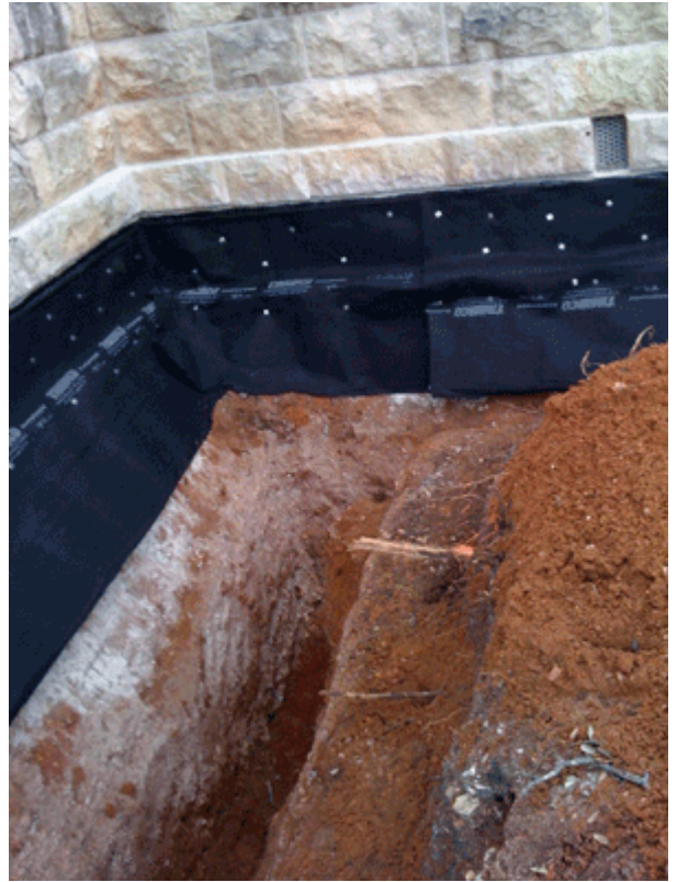
Drainage mat installed to cover waterproofing membrane material.
