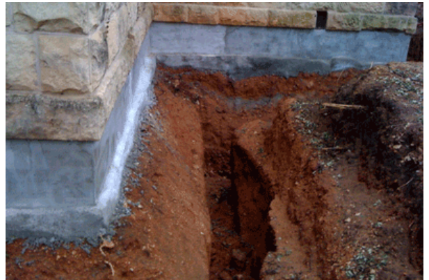
Parge coat applied to foundation footing.
