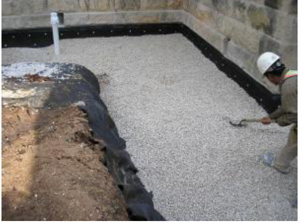
French drain filled with washed gravel
