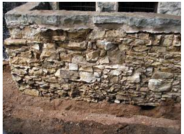
East Wall Exposed and cleaned
