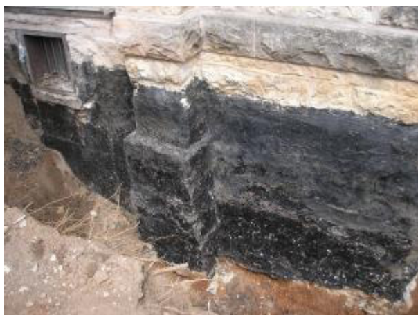
Existing tar waterproofing material
