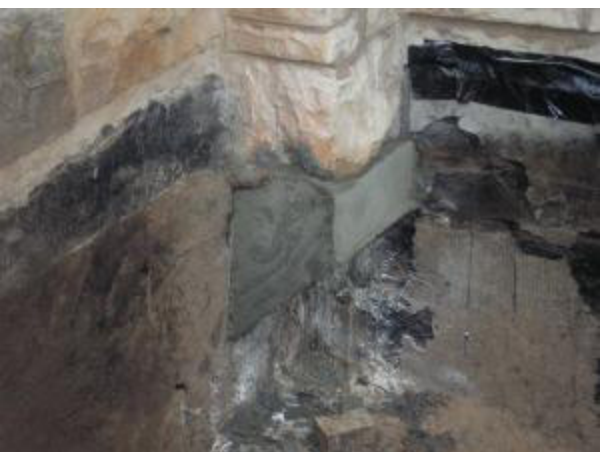
Under pinning of column
