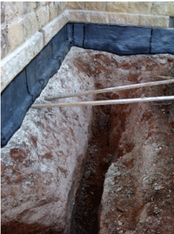
Waterproof membrane installed onto parge coat.
