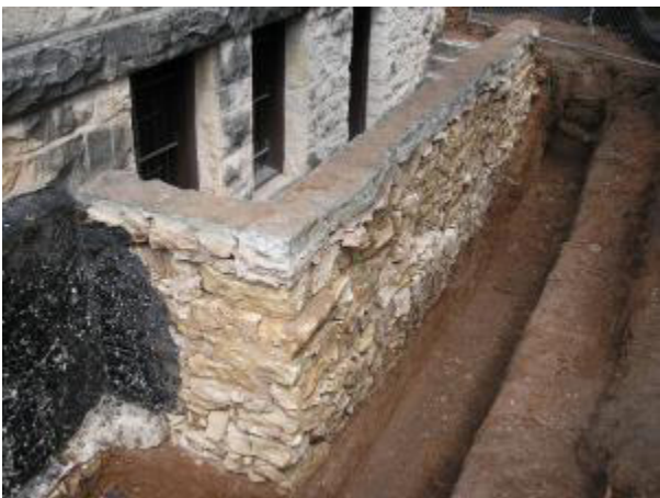
East wall excavated
