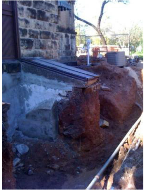
Underpinning of damaged hatch
