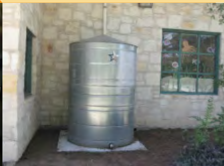
Zaragoza Recreation Center Rainwater Collection
