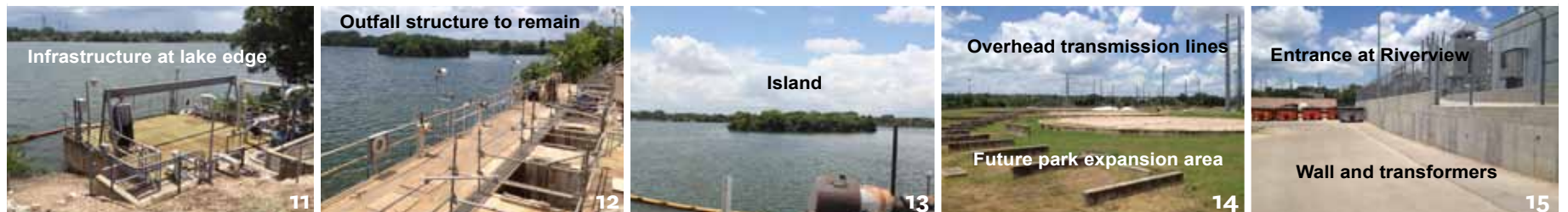
Figure 7. East Park Existing Conditions Observations
