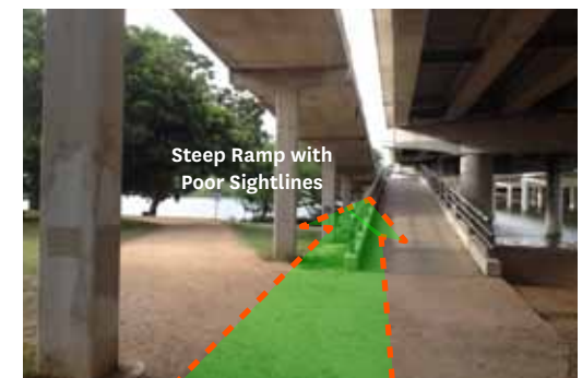
Figure 73. Pedestrian Bridge Next to IH 35 Existing View
