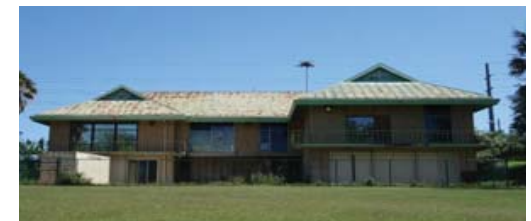
Figure 80. Nash Hernandez Building Existing View from Terrace
