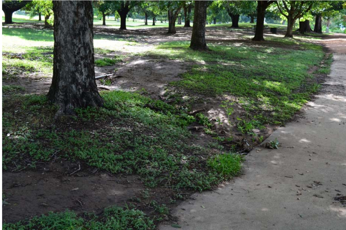
Erosion from parking lot, sediment is carried over jogging path and deposited into Lady Bird Lake directly impacting water quality.
