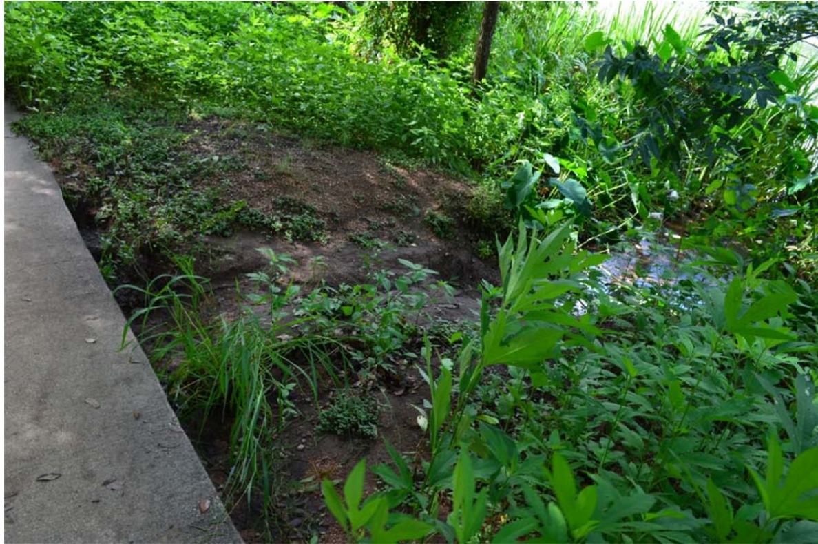
Erosion from upland area and parking runoff.
