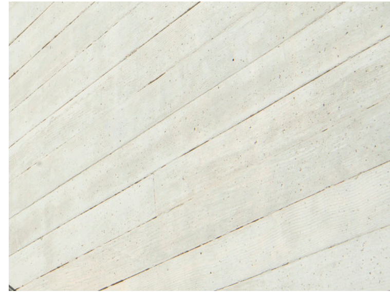
BOARD FORM CONCRETE
