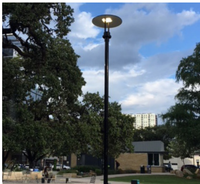
Recently-installed full cut-off pedestrian light fixture at Republic Square (Limbacher Godfrey Architects)
