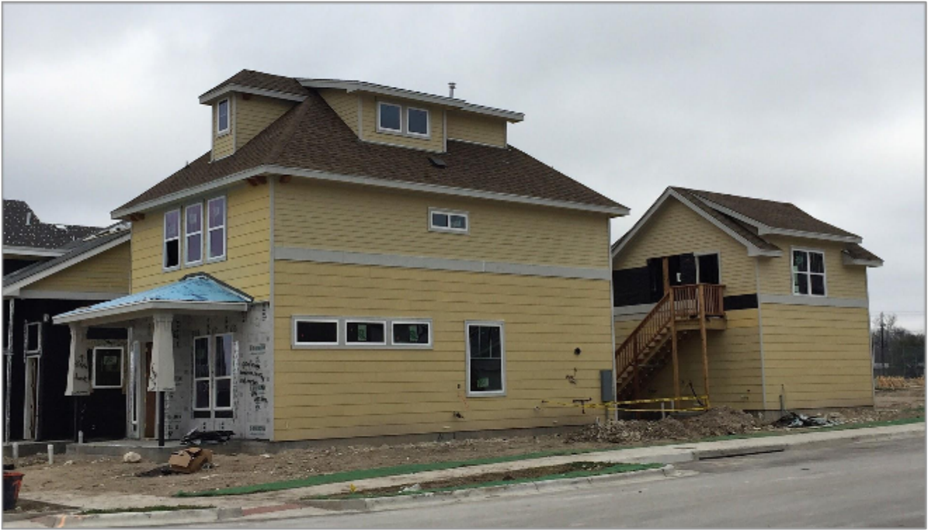
Single family home with garage apartment under construction in Crestview Station. Note the 10 ft. separation between the main house and the garage.
