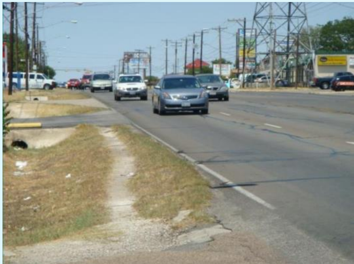
Sidewalks and drainage were not constructed with roadway or adjacent development
