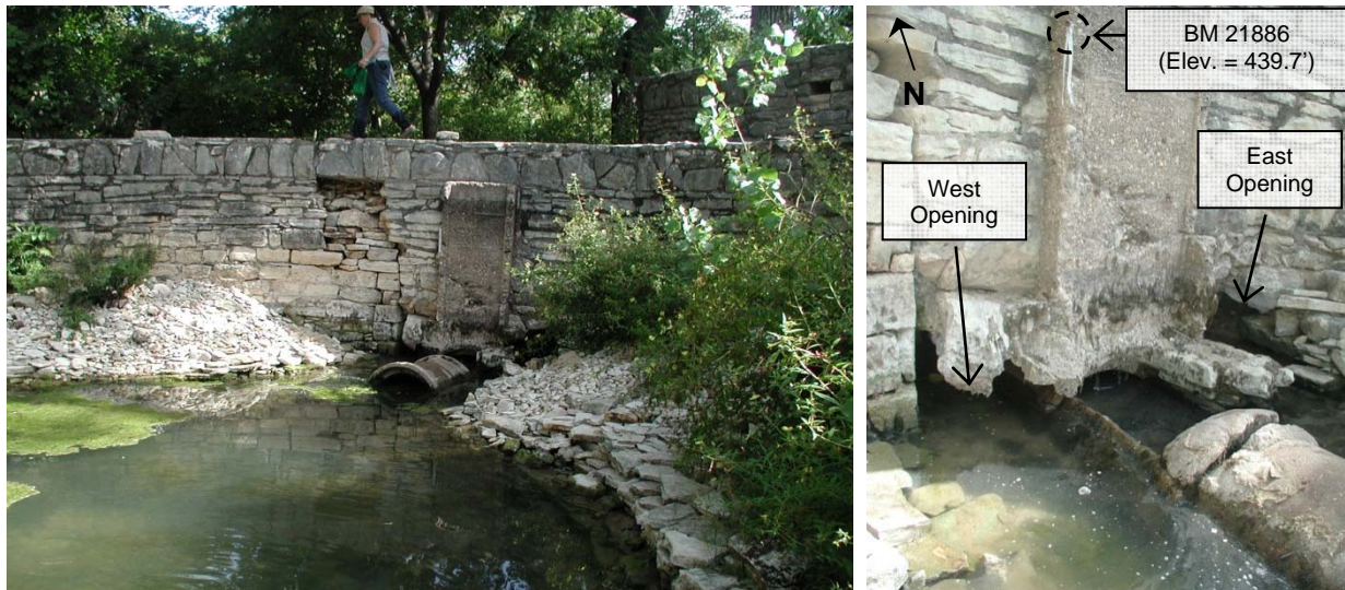
Figure 2.1.1: Outflow Exit Location – Views from within Enclosure Overall View (Left) and Close-up of Wall Openings (Right)
