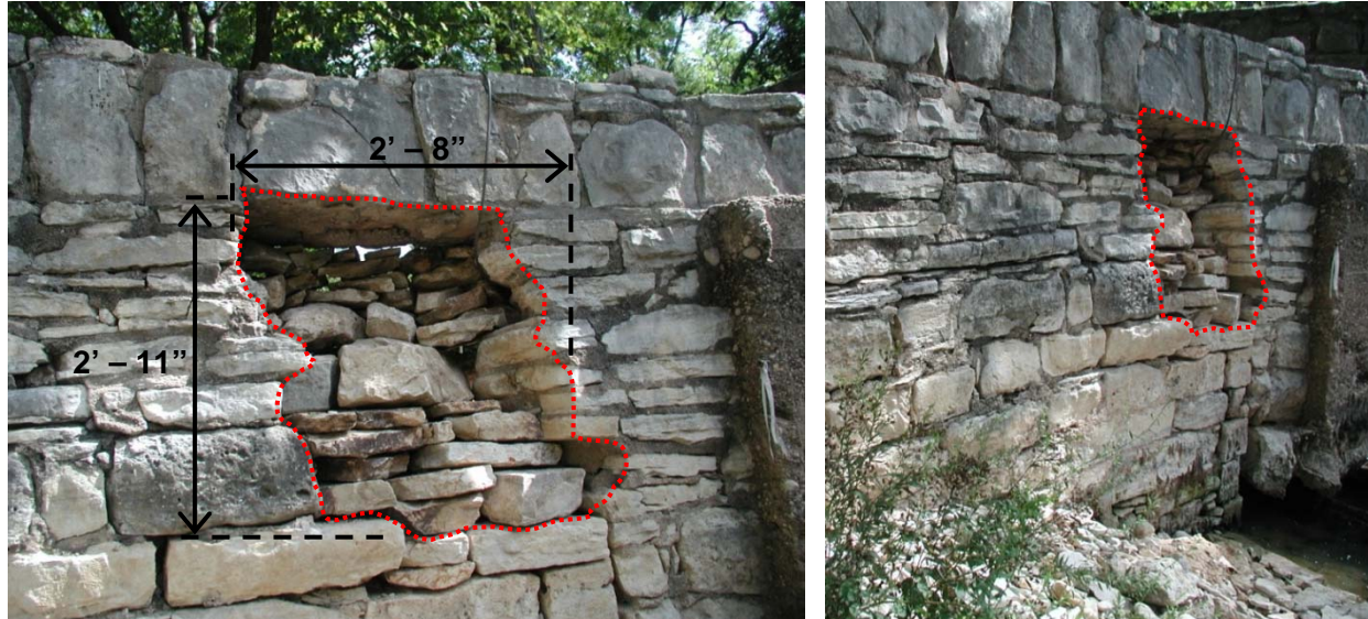
Figure 2.1.5: Portion of Wall with Dry-Stacked Rubble – Views from within Enclosure Straight-on View (Left) and Oblique View (Right)
