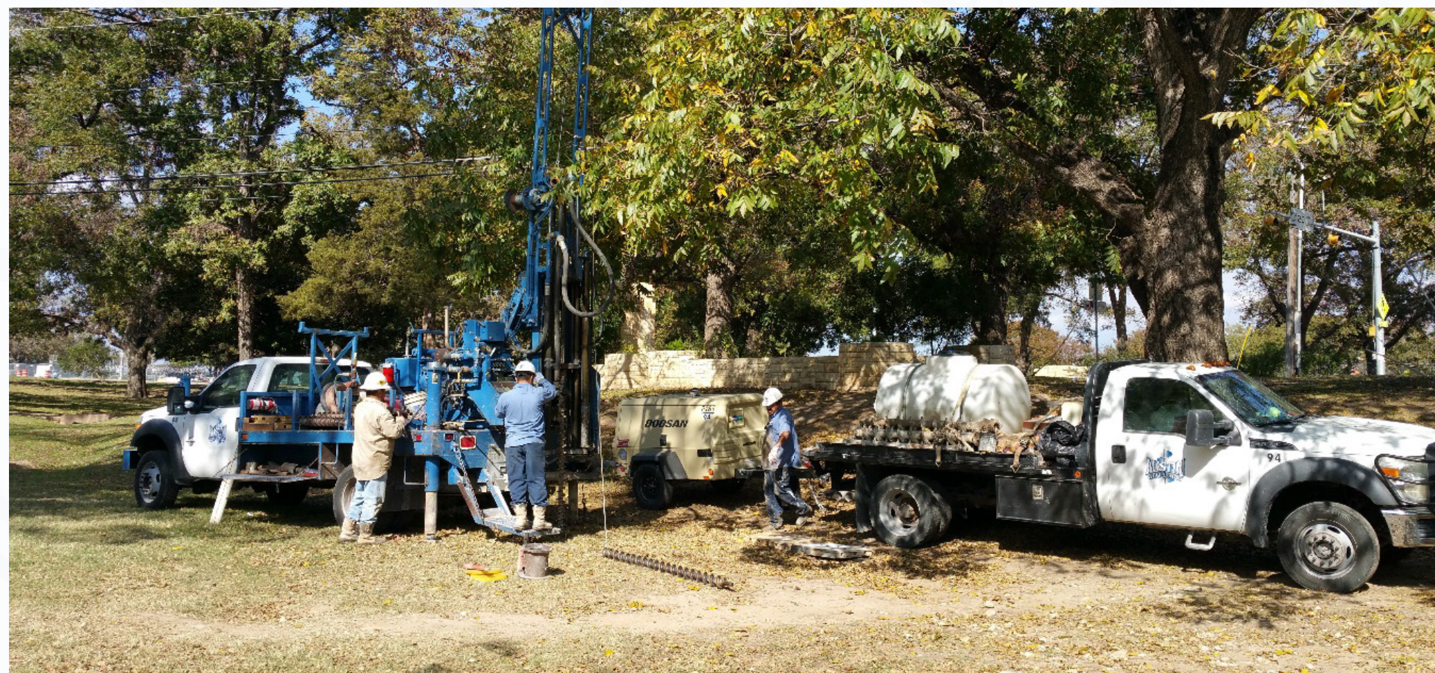
Geotechnical Borehole Drilling for subsurface conditions
