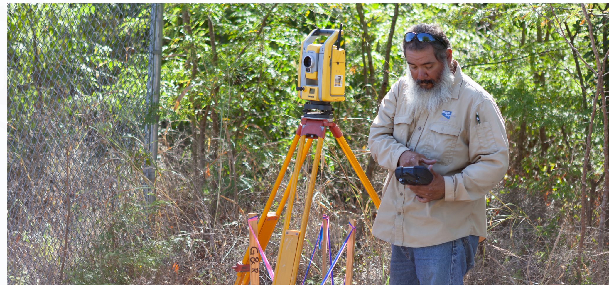
Survey Crews to identify topography and existing conditions
